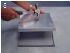
5 After screeding is cured, use a hammer & gently remove the disposable lid
