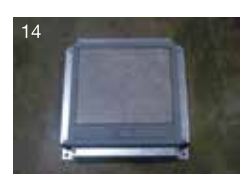
14 If tile is thicker than the recess, grinding is necessary. Remove the throw-away lid and install the frame & trap
