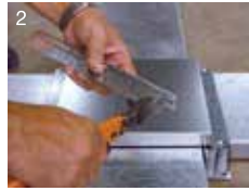
2 Cut off the pre-punched knockouts at the side blank plate
